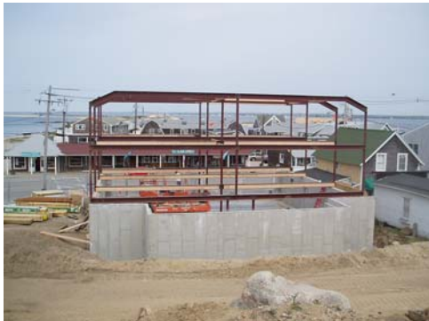
Concrete walls and steel moment frames
