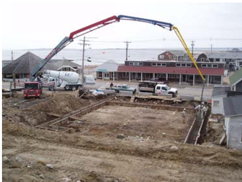
Installation of perimeter grade beams on piles
