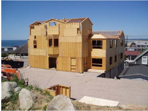
Wood framing in progress
