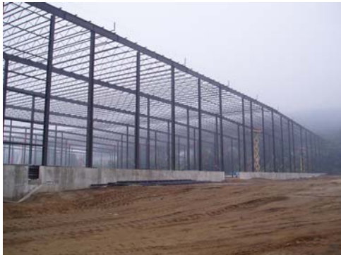
Steel framing nearly complete
