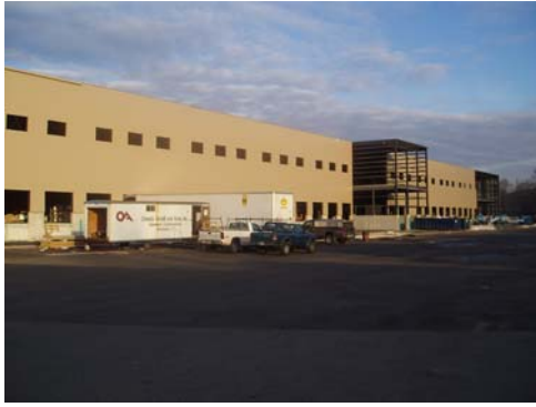
345,000 SQFT addition to distribution center
