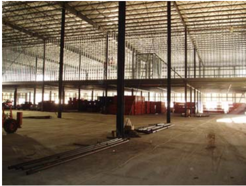
Open interior with mezzanine
