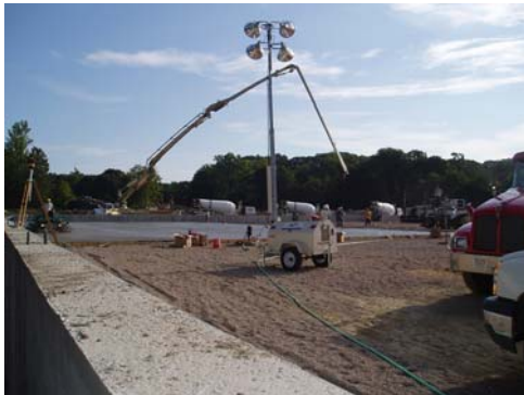
Installation of high performance concrete slab
