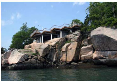
Cantilevered pool deck in Stony Creek, CT
