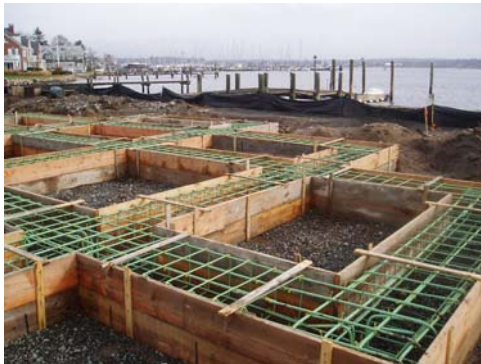
Concrete grade beam foundation on piles
