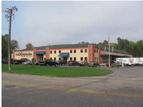
Renovation for SECONN Warehouse
