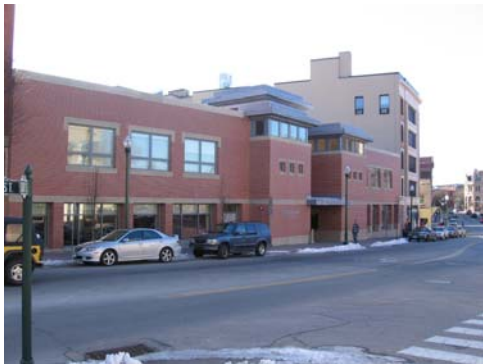
Renovations to Otis library
