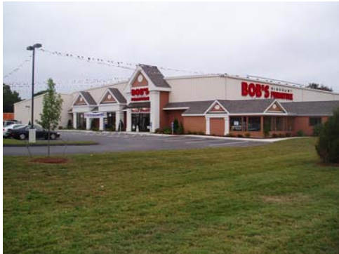
Renovations to Bob's Discount Furniture
