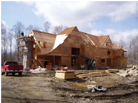
View of building under construction
