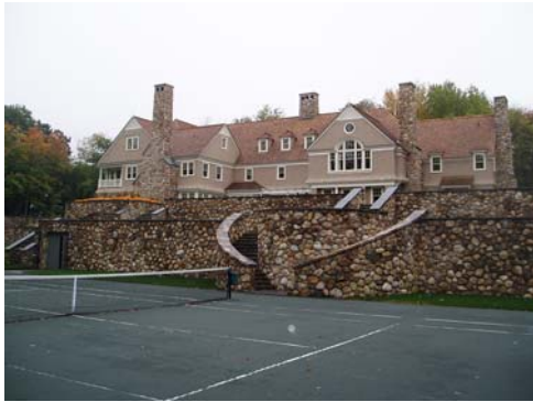
Various levels of site retaining walls
