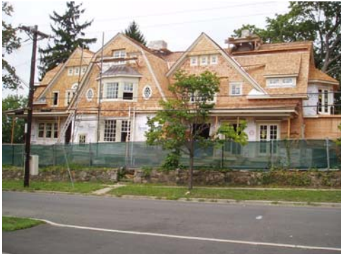
Installation of roofing and siding
