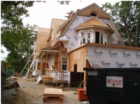
View of building under construction
