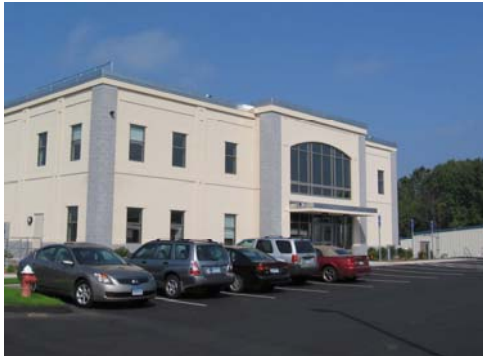
ABCO Welding Headquarters, Waterford, CT
