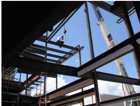
Steel framing at towers near entry
