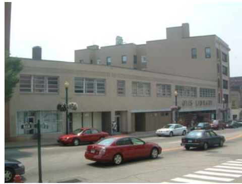
Front of building before
