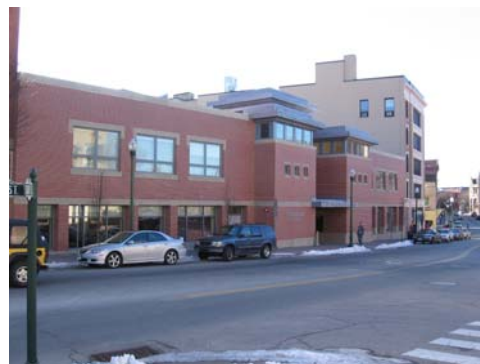
Front of building after
