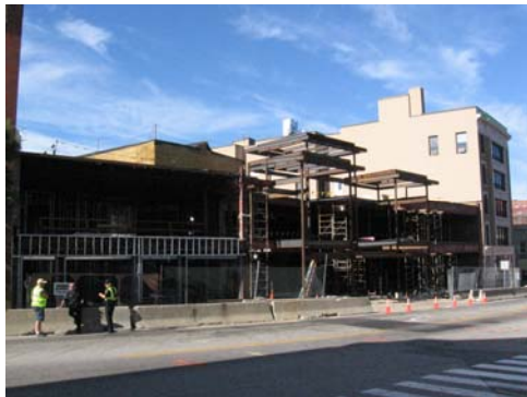
Steel tower framing at the front facade
