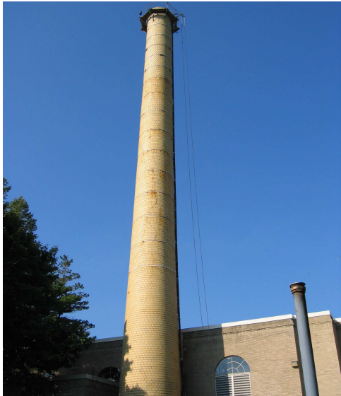
Connecticut College Radial Brick Chimney
